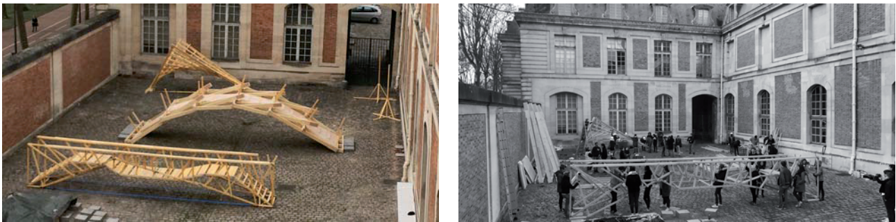
Fig. 2. Constructed Bridges - Domestical Wildness, Triangle Reciprocal Structure, Hyperboloid Paraboloid
