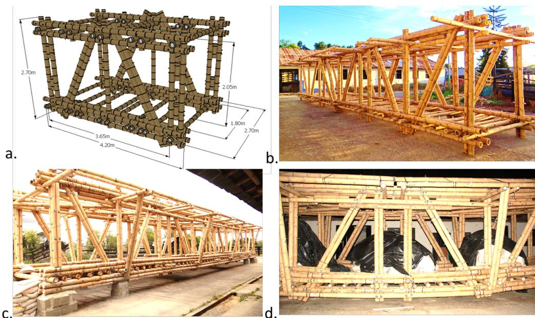
Fig. 1. Modular bridge a. Proposed model, b.,c.Real scale prototype of the bridge, d. Load Test
