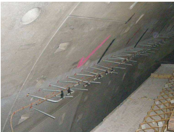
Fig. 1: Post-installed reinforcement
