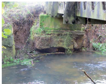
Fig. 1. Extent of scour at abutment
