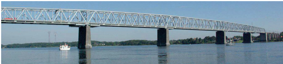
Fig. 1: Overview of the railway bridge across Little Belt, the only railway link between the western and the eastern part of Denmark. The 4 main piers are situated in seawater, 60 m from the seabed.
