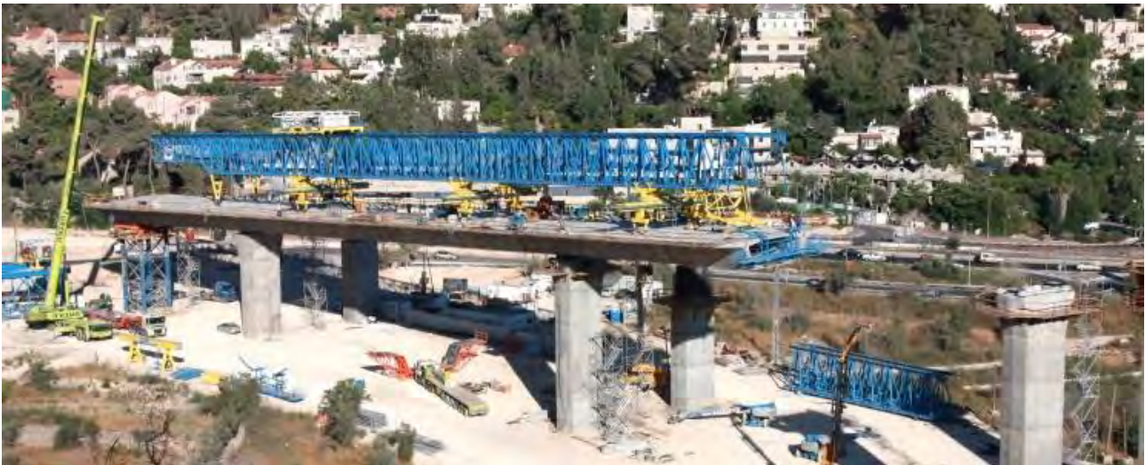
Figure 1: Precast segmental bridge under construction, using overhead launching gantry (Jerusalem, Israel)
