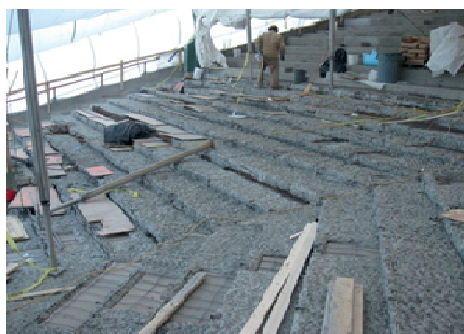
Figure 1. Demolition and surface preparation of seating riser section.
